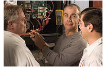
Gerry Rodino (center), training coordinator for Calvert-Jones, provides some chiller training tips to Norman Carter (left) and Chris Ward, both field supervisors.
